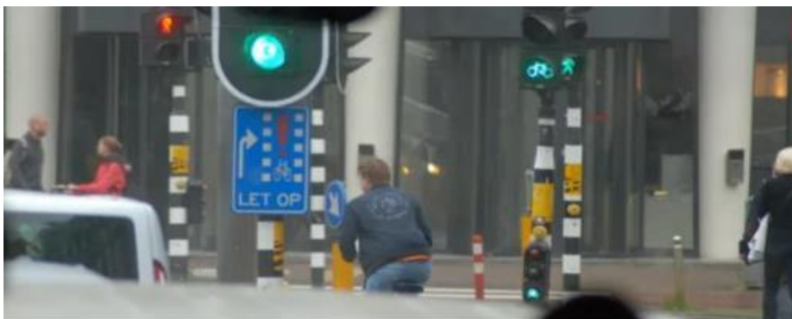
Figure 2.56 Example from the Netherlands of traffic signals + give way signage controlling turning traffic and cyclists (Source: Dutch Design Guide Ontwerpwijzer Fietsverkeer)
