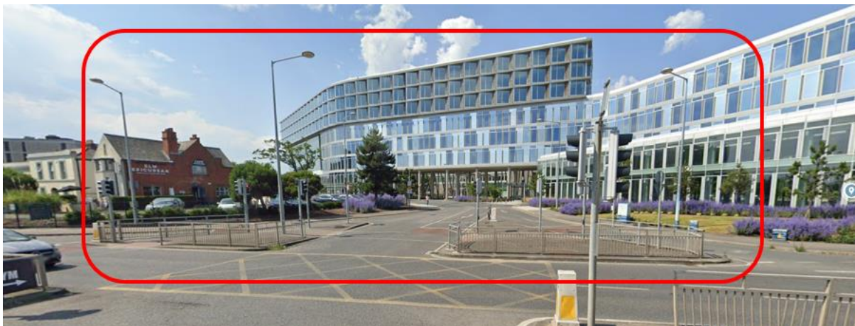
Figure 3.46: Existing Street View at Elmpark Green Merrion Road (Image Source: Google)
