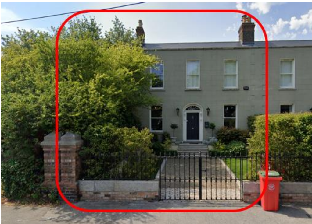
Figure 3.75: Existing Street View at (Image Source: Google)
